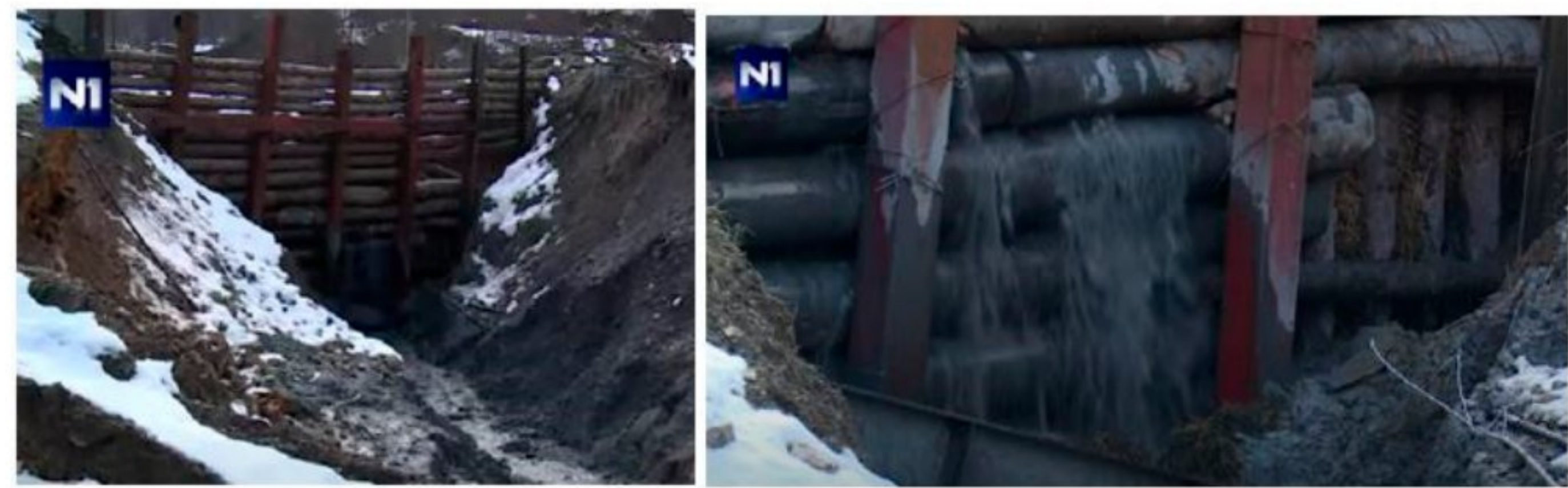
Figure 7. The temporarily blocked eastern tailings field was breached again on 17 July 2014. Reproduced with permission from N1 Television [19].
