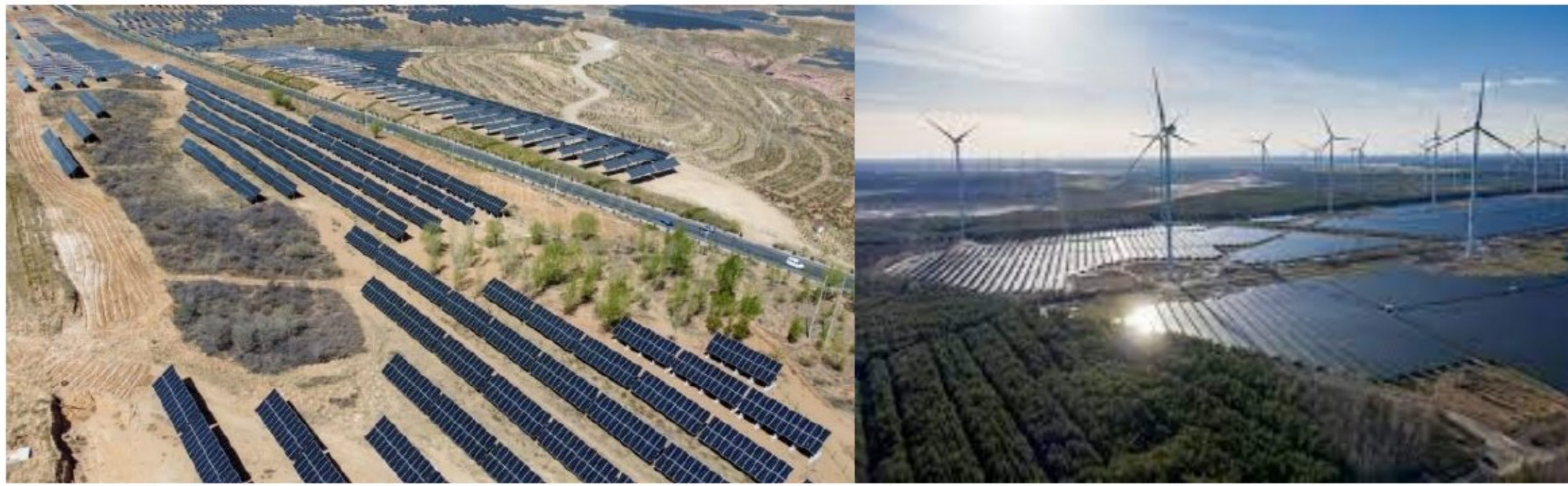
Figure 3. Using solar and wind energy on recultivated site - Photovoltaic panels in Boortai Coal Mine in China (2022) on left side, solar plant in Klettwitz, Germany on right side
