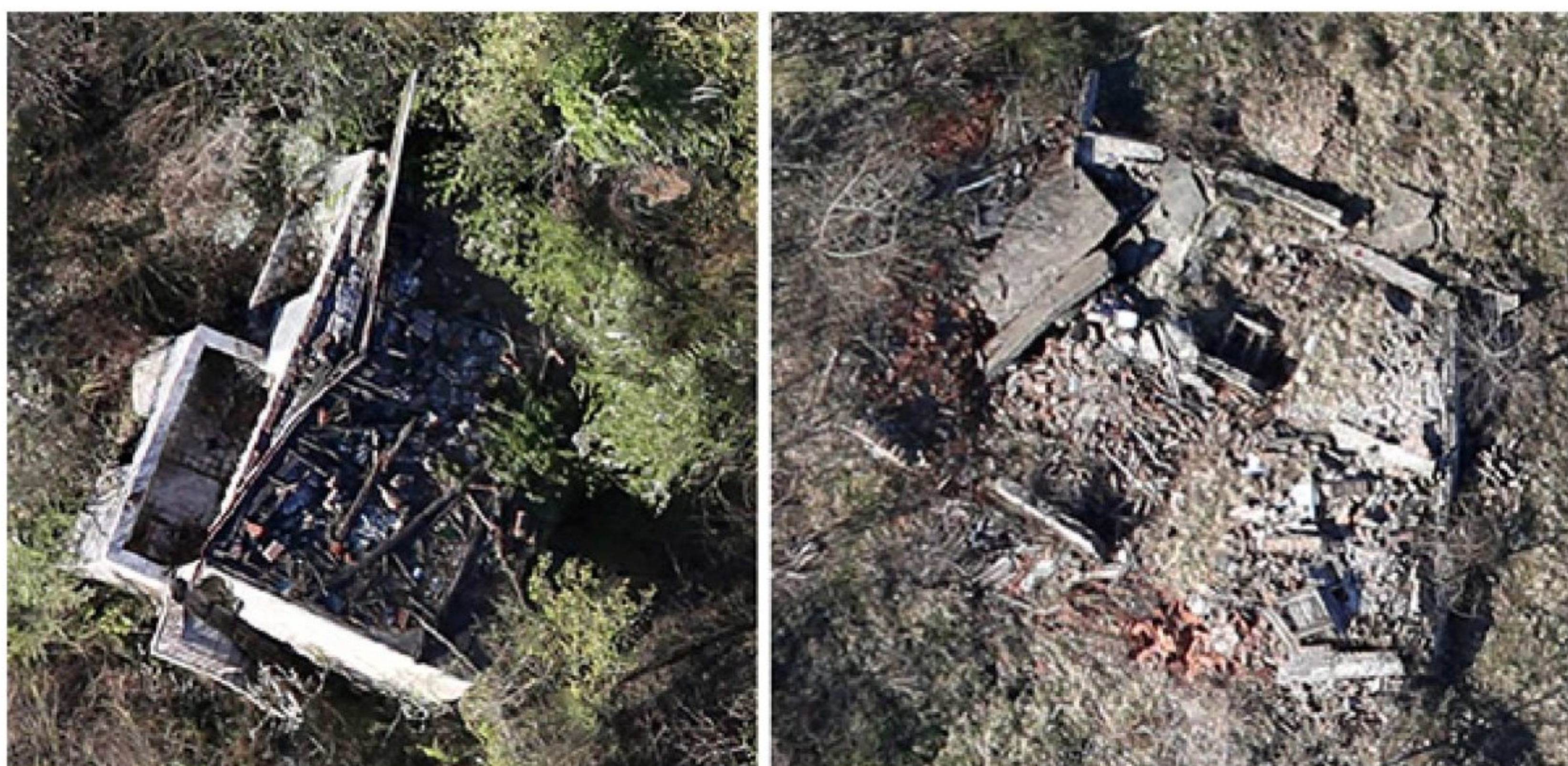
Figure 3. Aerial images of two destroyed buildings on the 'Umka' landslide that are inaccessible and surveyed by UAV remote sensing.
