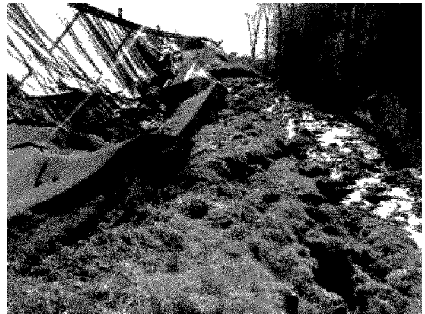
Figure 4 Main scarp of the Dubravci landslide.
