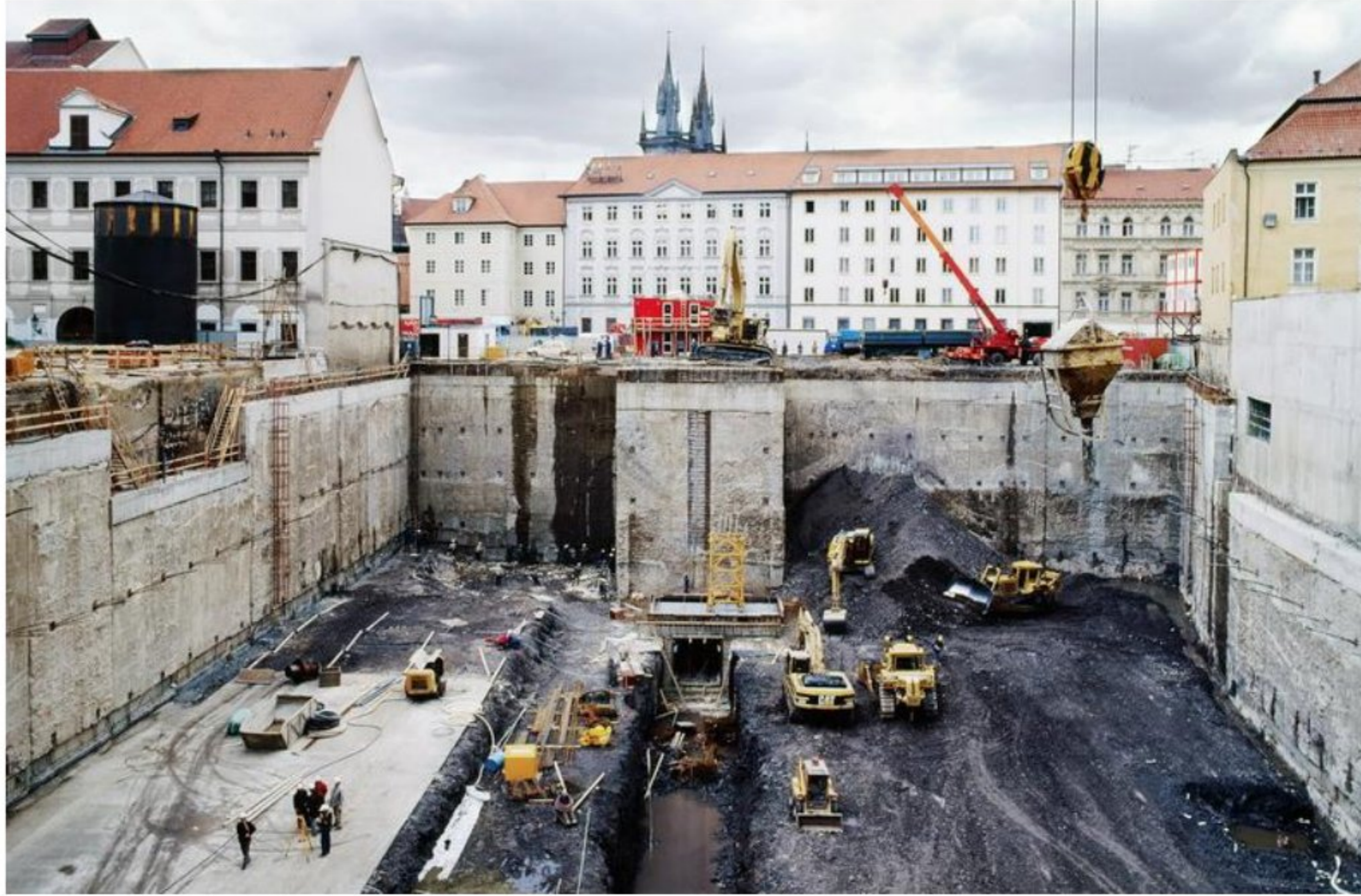
Figure 1 An example of excavation of rock material in an urban area (Zakladani, 2023)
